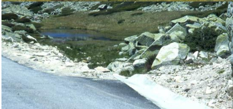
Figure 18 Top: Menyanthes trifoliata , Southern damselfly ( Calopteryx xanthostoma ). Mid: bog polluted by plastics used by “ski-tourists”. Bottom: gutter along the road made of allochthonous calcium containing material (concrete) discharges in bog system. In winter large amounts of salts used for road gritting flow in the system, raising the conductivity of the extremely soft waters.
